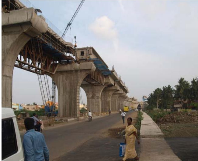
MRTS Phase II extension project in progress
