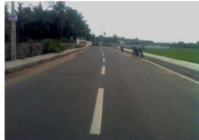
Widening and Strengthening of Madharvedu road under TNUDP III
