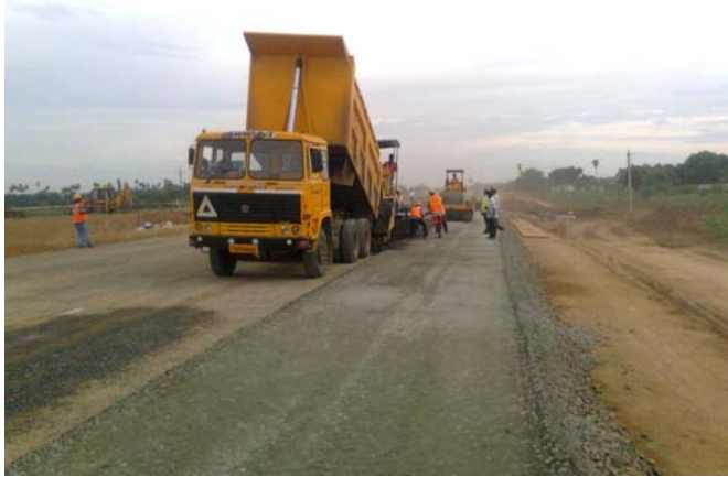
Phase I Outer Ring Road project in progress
